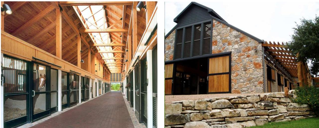
Oakhaven Ranch – Austin, Texas – The installation of translucent surfaces in the roof allow the heating of the air in the upper part of the stable, creating the correct natural air circulation. A good number of opened surfaces, correctly positioned, allow natural air circulation (stall doors, windows with fins on the roof and on the upper part of perimeter walls.) (from J.A.Blackburn – Healthy Stables by Design)
